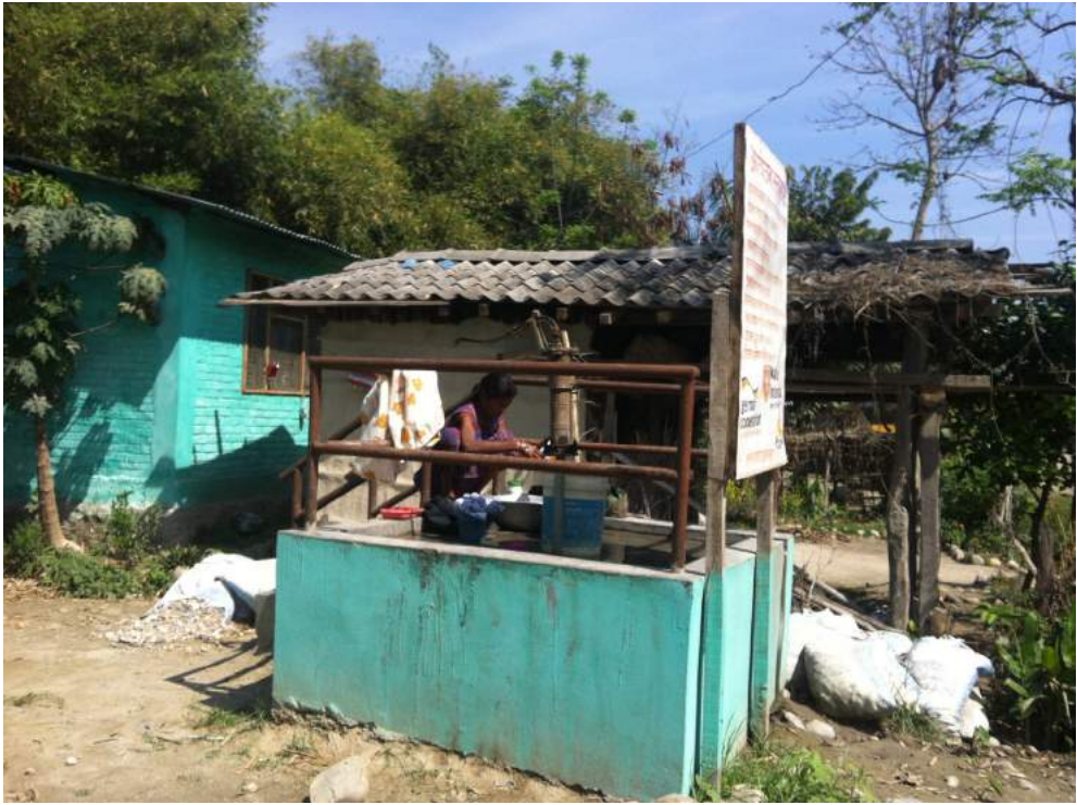
Figure 3.3: A raised water pump in a case study wards in Bardiya.
